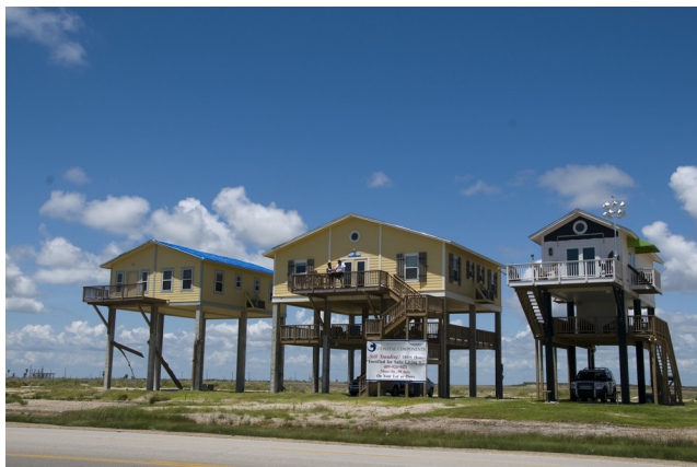
FIGURE 1-1 Gilchrist, Texas, August 16, 2009. These stilt homes were the only structures still standing in the town of Gilchrist after Hurricane Ike destroyed it. FEMA is still working with local, state, and federal agencies to rebuild the town. Photo by Patsy Lynch/FEMA.
